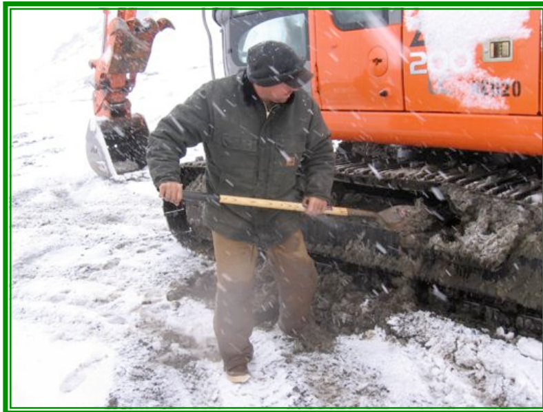
Figure 3. Challenging weather, August 19, 2006.
