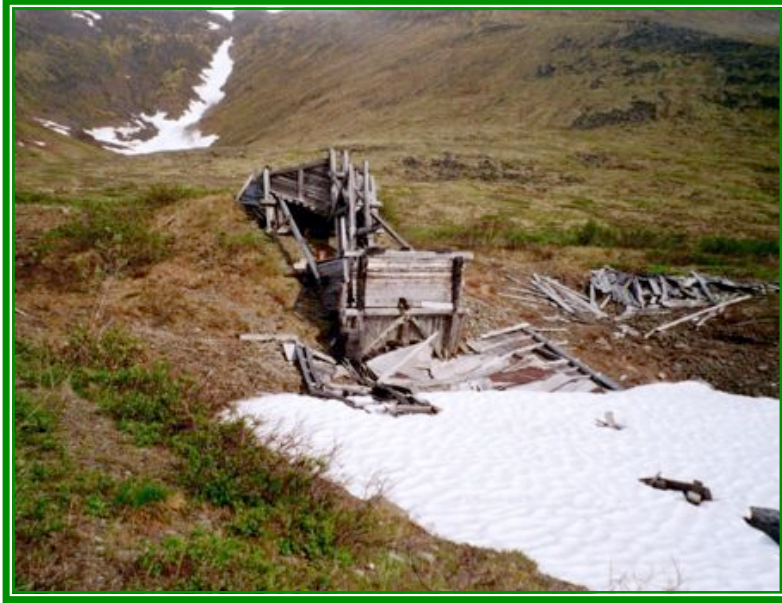
Figure 27. The Touissant Mill ruins and the prospect area of the Indicate-Tonapah veins.
