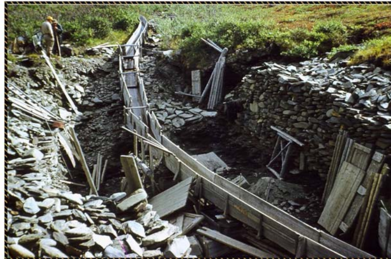
Tobin Creek sluice box as it appeared in 1961. Note: hand-stacked boulders on the right.
