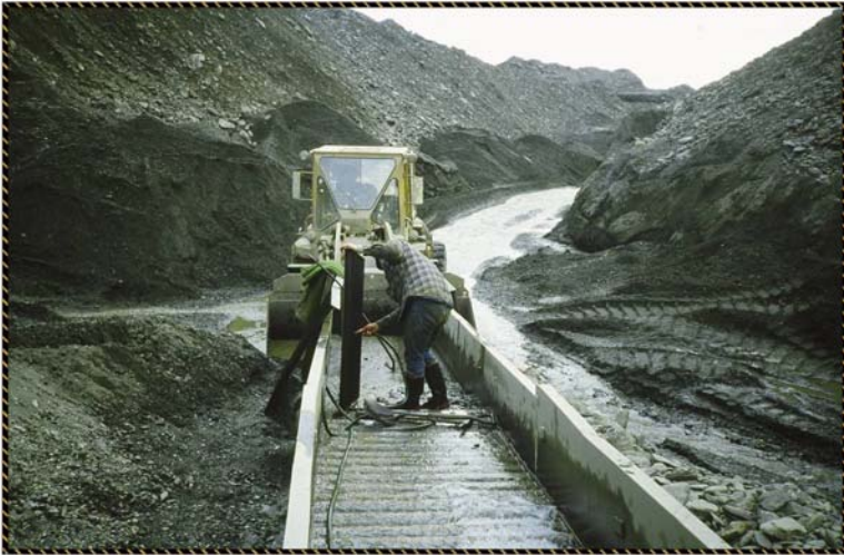
Tobin Creek placer sluice box maintenance and repair, August, 1986
