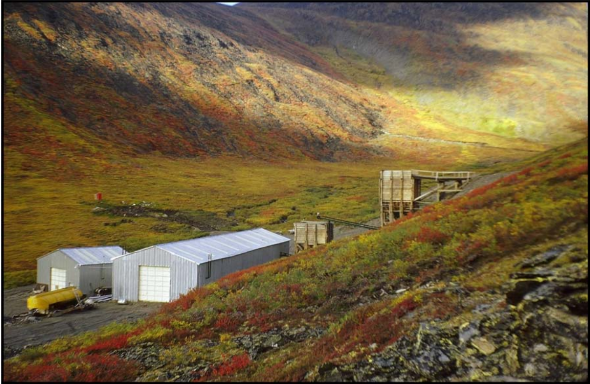
Figure 27. Photograph of the Tobin Creek 100 ton per day mill.
