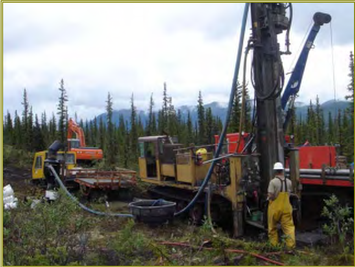
Figure 21. Conventional reverse-circulation drilling system.
