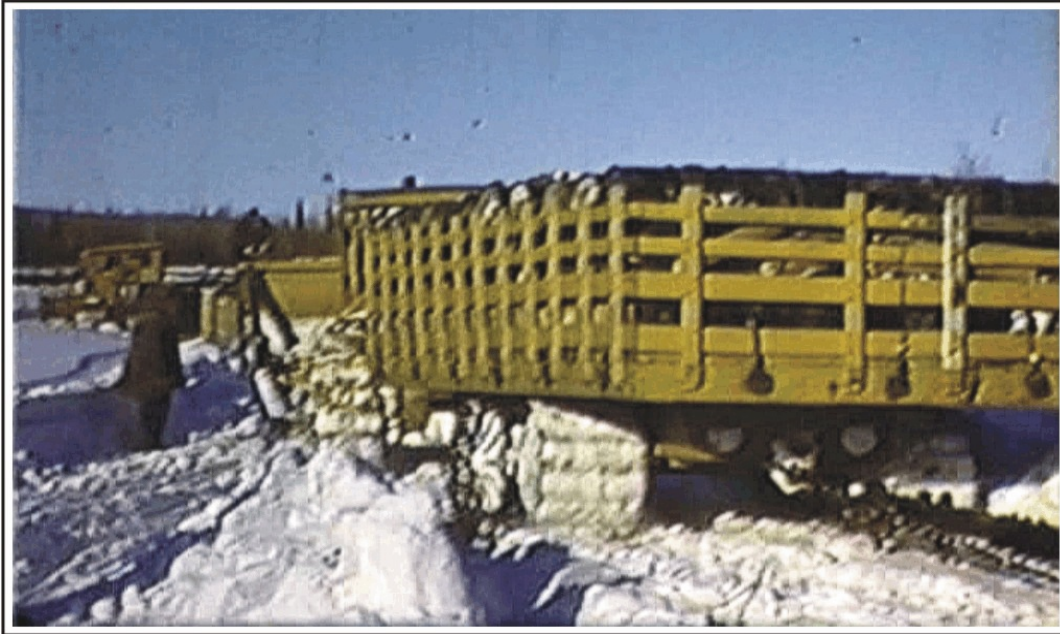
Figure 22. Repo and Schwaesdall cat-train en route to Myrtle Creek on the east end of the Caro-Coldfoot and Coldfoot-Chandalar trails, spring 1939. The tracked trailer carrying fuel barrels is being pull by a tractor. The lead tractor (far left) is also pulling a trailer. Photo reproduced from “2006 Placer Mining Convention Film,” courtesy of George Lounsbury, Fairbanks.
