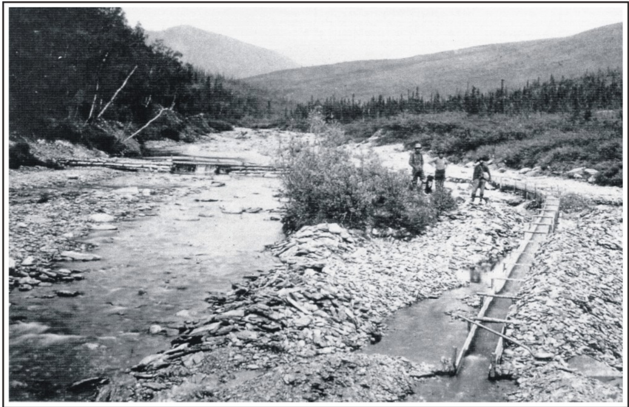
Figure 5. Placer mining on Myrtle Creek in 1899, the first major gold discovery in the Koyukuk Mining District. Photo by F.C. Schrader, U.S. Geological Survey, Denver, Colorado.
