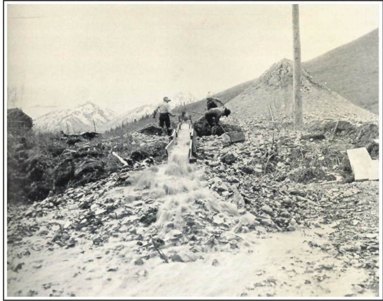
Figure 24. Sluicing winter gravels from a drift mine, early 1930s. Photo reprinted from Robert Marshall, Arctic Village (1933), p. 161.
