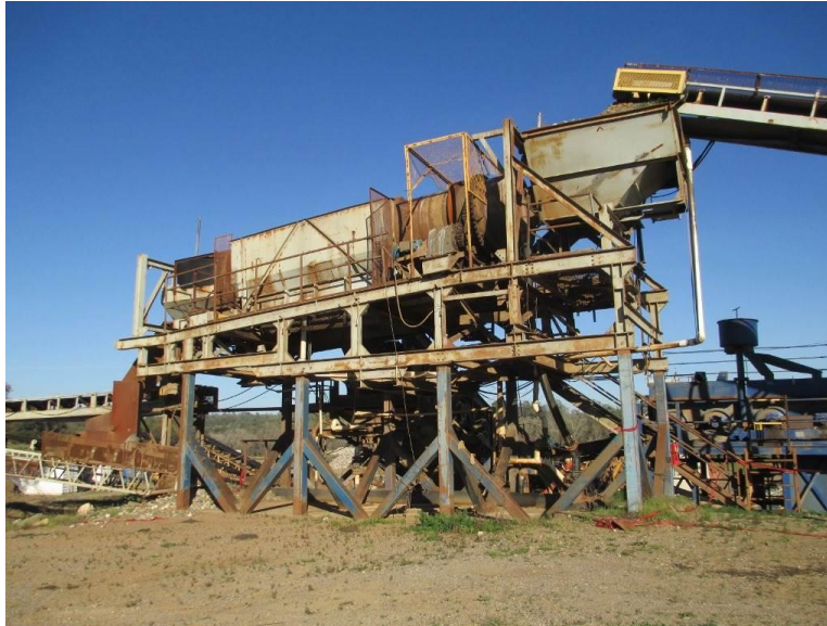
Photo 17-1: Typical Trommel Gold Recovery System
