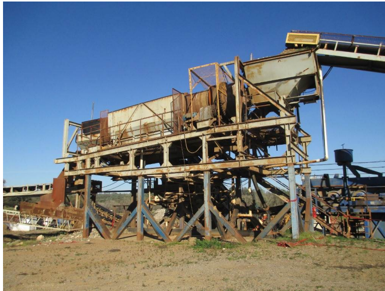
Photo 17-1: Typical Trommel Gold Recovery System
